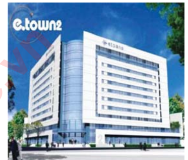
E.Town 2 Building, HCMC 6 Passenger lifts 1600 - 2000kg, 1.75 & 2.5 m/s
