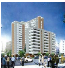
Nguyen Bieu Apartment, HCMC 10 Passenger lifts 750-1000kg, 1.5 m/s
