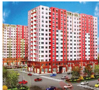
Thai An Apartment, HCMC 5 Passenger lifts 800 - 1600kg, 1.75 m/s
