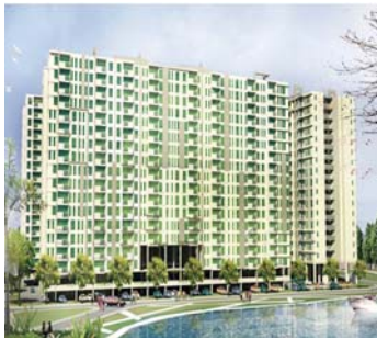
An Phu - Binh Khanh Apartment, HCMC 10 Passenger lifts 1600 & 2000kg, 1.75 m/s
